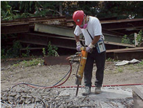
Jackhammering with a water spray control that reduces dust.
